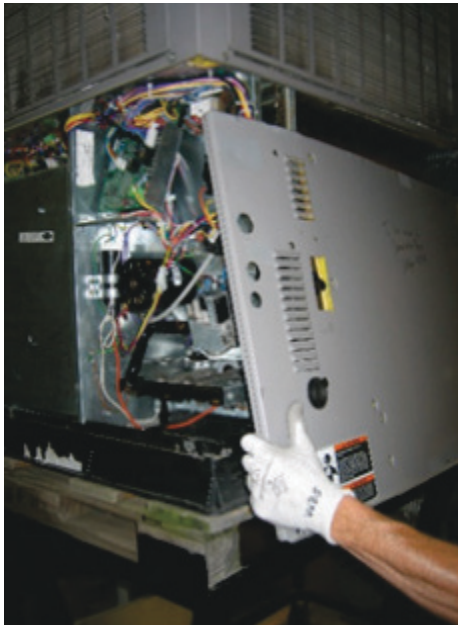
Fig. 34 – Replacing Right Side Panel
